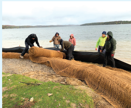
A woven coir blanket is draped over the sand slope, coir log, and large toe stones are placed in a trench to form the base of the slope.
