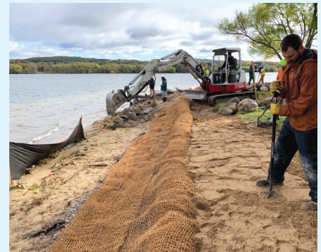
A woven coir blanket is draped over the sand slope, coir log, and large toe stones are placed in a trench to form the base of the slope.
